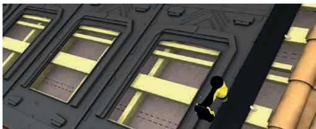
Pre-drilling of GSE frames + flashings + edge wedges
